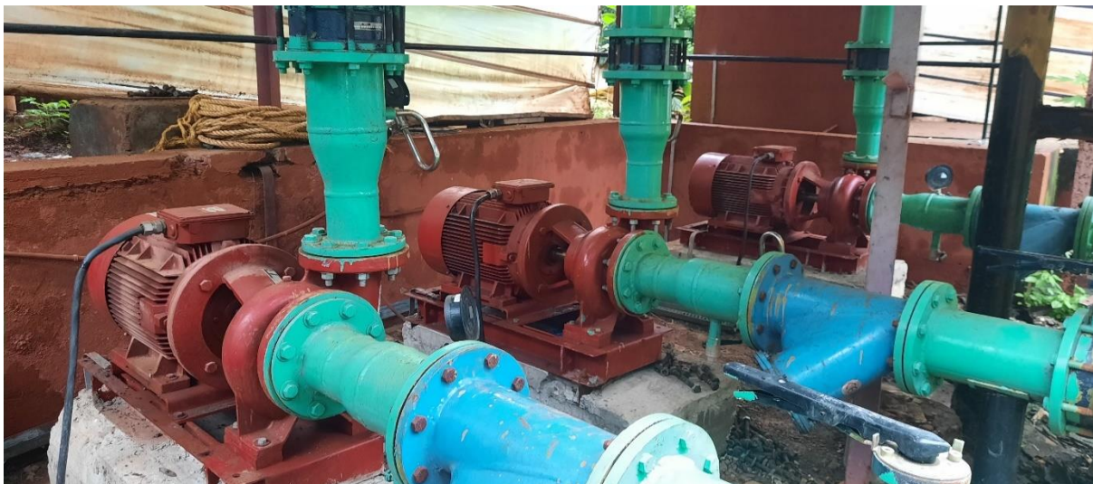
Figure 4: Condenser Pumps
